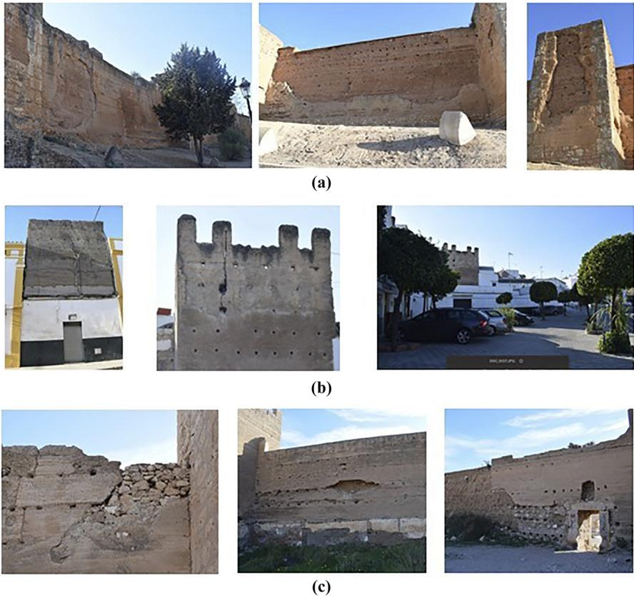
**Figure 5.** Detachment, fractures and erosion processes identified: (a) Niebla; (b) Marchena; (c) Almería
