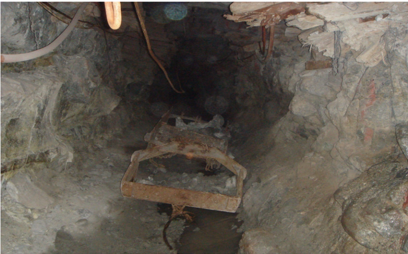
Figure A12: Scraper-Winch with Which to Remove the Broken Rock
